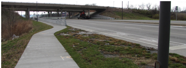
Existing 210 and Chouteau Trafficway Intersection, Looking South
