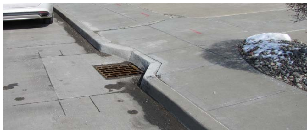
FIGURE 1.12 EXISTING CONDITIONS ALONG THE BURLINGTON CORRIDOR
