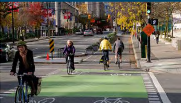
Buffered and protected bike lanes bicycle tracks provide a safe environment for bicyclists.
