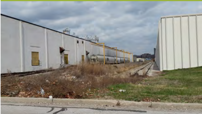
Abandoned railroad spurs create opportunities for future alley connections.
