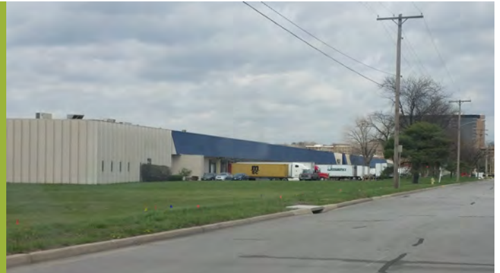
Adaptive reuse of buildings is encouraged to enrich additional activity in the surrounding area.
