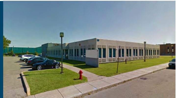
Landscape buffer and sidewalks enhance look and feel of area.
