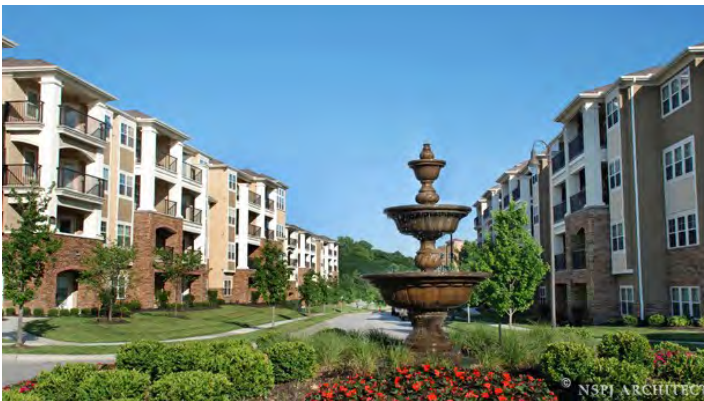
Multi-Family Housing. The Briarcliff City Apartments in Kansas City, MO. Landscape features, sidewalks enhance neighborhood.
