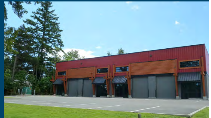
Enhanced warehouse buildings can add character to area.
