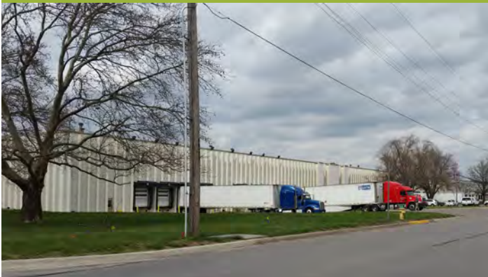
Provide landscape buffer to improve appearance of loading areas and public-rights-of way.
